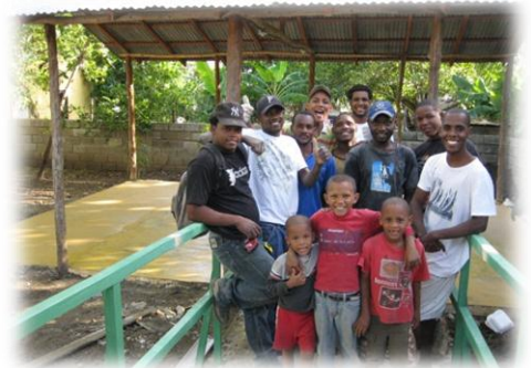
Group Home backyard – ramp and outdoor shelter completed
